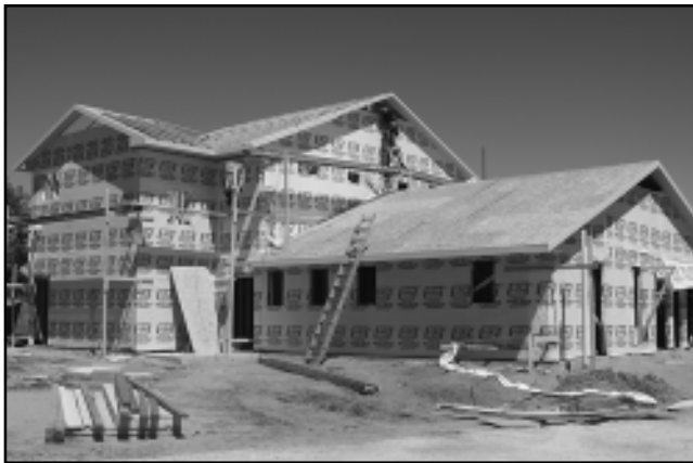
The Pit Stop is nearing completion!
